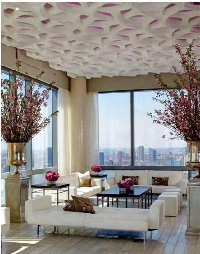
OPEN GRILLE LOOP CEILING WITH ACOUSTICAL PLASTER
