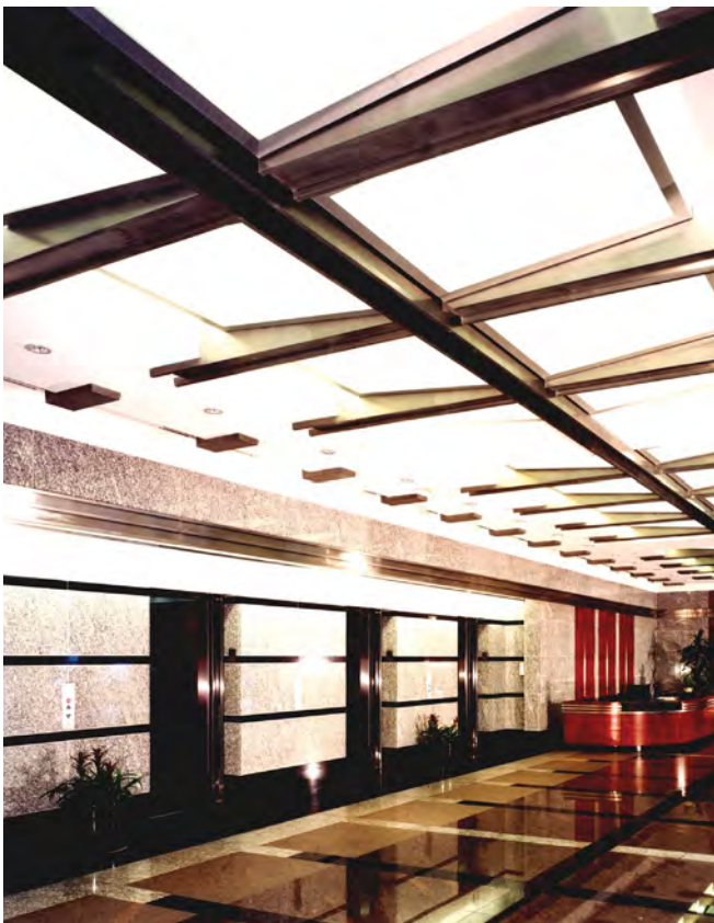
CEILING BEAMS AND BRACKETS
