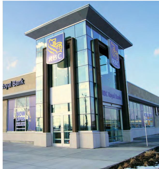
CORNICES & PORTAL ENTRY
