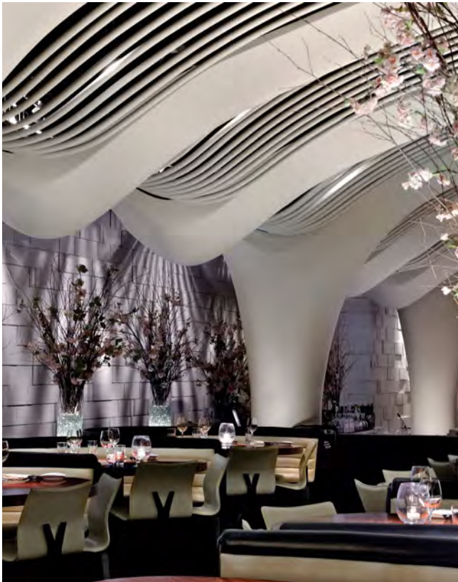
GFRG CONTOURED COLUMNS, CEILING FINIS, 3D WALL PANELS
